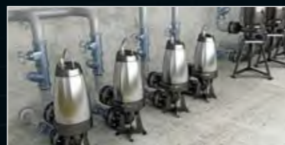
The SEV-SE1 pumps are suitable for vertical or horizontal installation to suit specific application arrangements.
