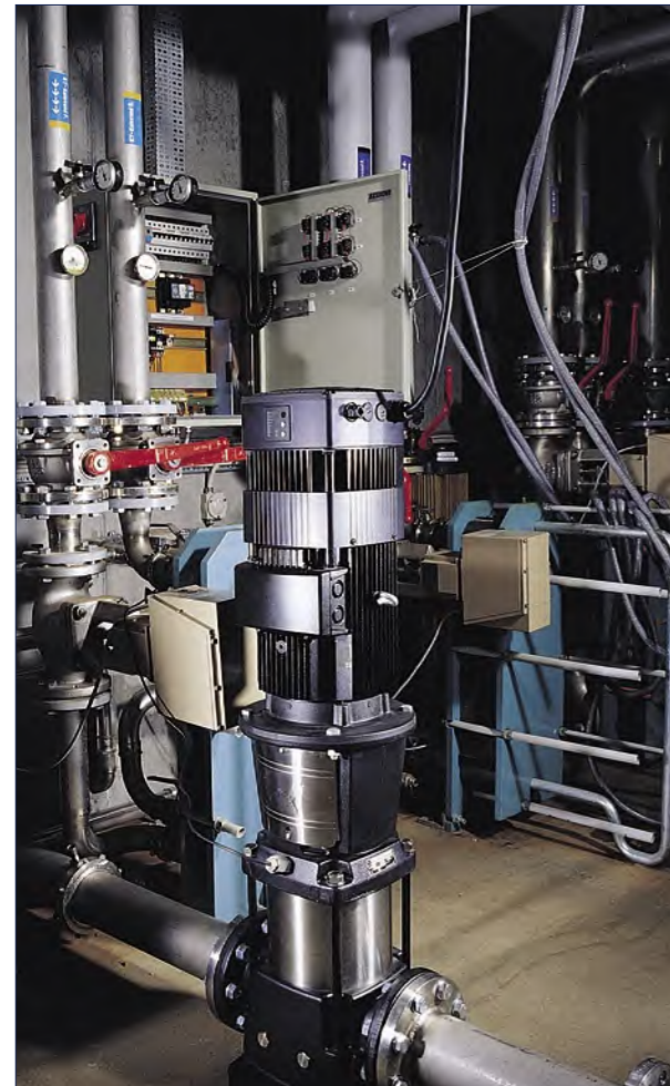
The CRE pumps represent a happy union between high-quality pumps and superior variable-speed motors. Here, a variable-speed motor is used to give the final touch.
