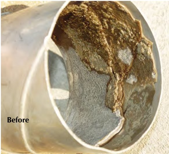
A piece of stainless steel from a bore pump; the scale build-up was up to 7mm thick and laminar in appearance.
