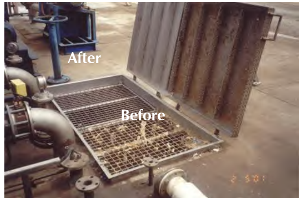
Cleaning of waste water pit covers.
